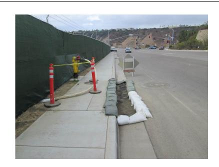
**Photo 3:** Check dams and inlet protection measures consisting of filter fabric were observed being maintained along Mira Sorrento Place in accordance with APM-HYD-1.
