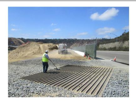
**Photo 4:** Trac-out measures consisting of a rattle plate and rock apron are being maintained at the construction site entrance in accordance with APM-HYD-1.
